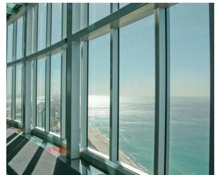
**DOUBLE GLAZING** - The system is versatile enough to accept both single and double glazing units up to 24 mm thick. Double glazing units, incorporating a 12mm airspace, give significantly better thermal and acoustic insulation than most other double glazed windows.
